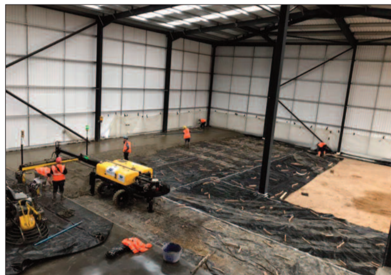
▲ The Level Best concrete flooring team working on a new warehouse floor slab in Reading.
