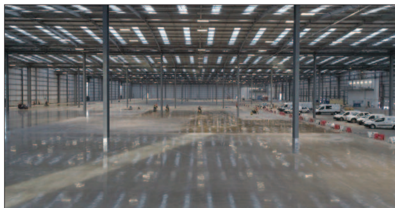
▲ In the foreground, FRS completed floors whilst works are ongoing in the background.
